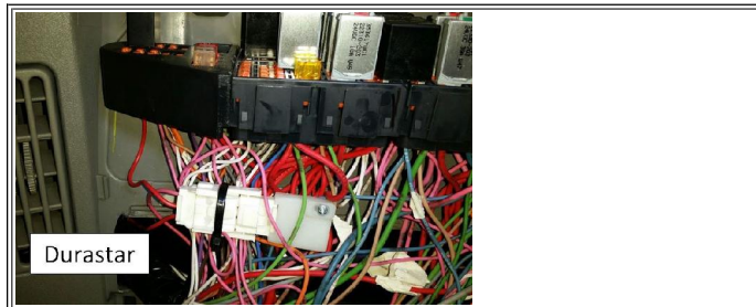
Figure 4: Rectifier Diode Inspection
