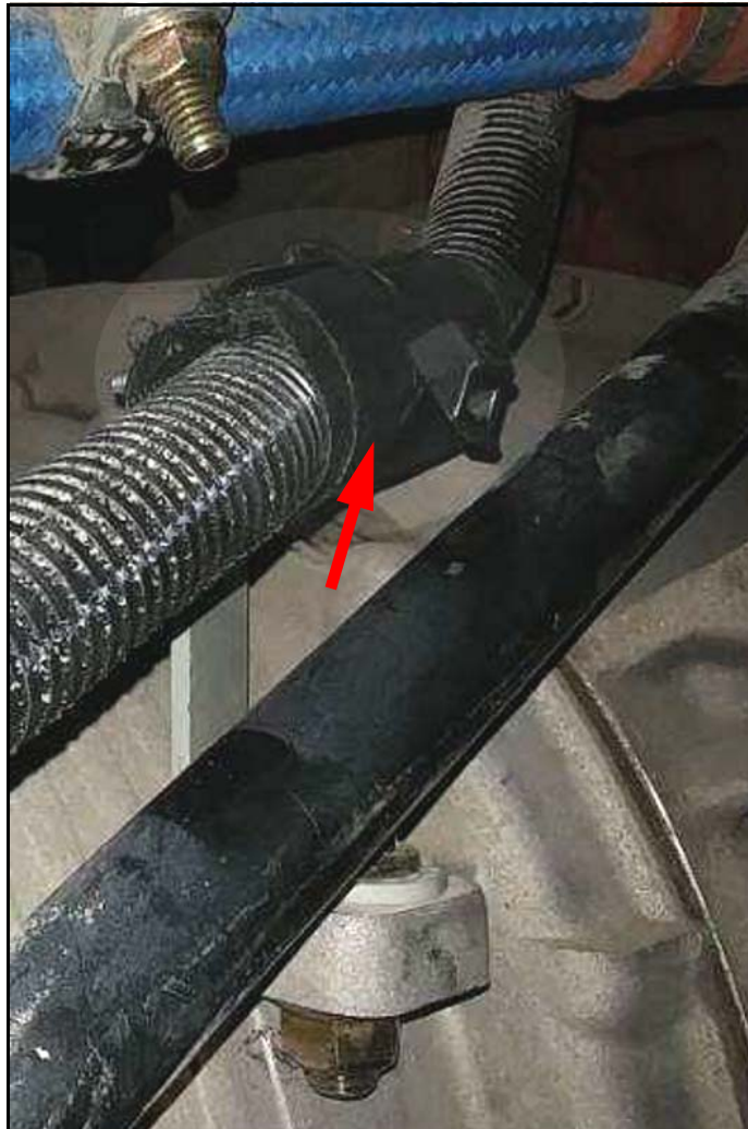
Figure 23. Installation of heavy duty wrap over the transmission harness.
