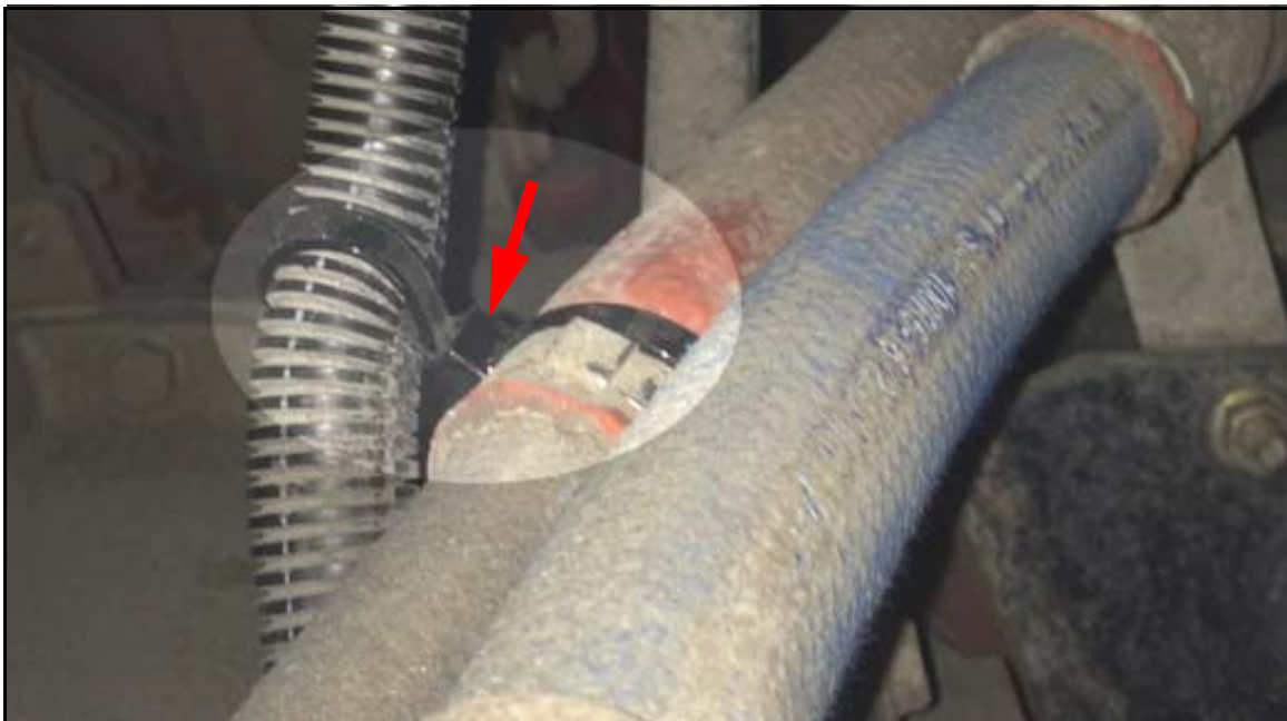
Figure 25. Double loop cable installed with base positioning.
