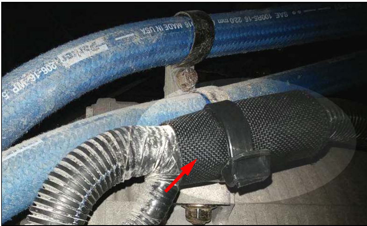
Figure 22. Installation of heavy duty wrap over the transmission harness.
