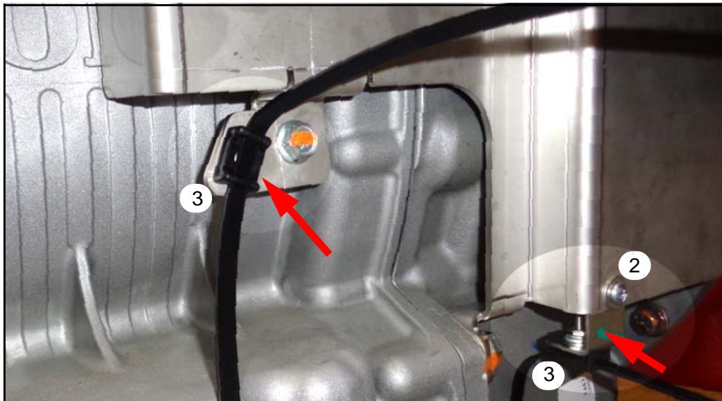
Figure 20. Bracket and tie base install on protection shield.
