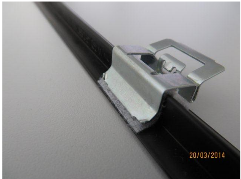
Figure 4: Retaining clip isolated with the fleece tape.
