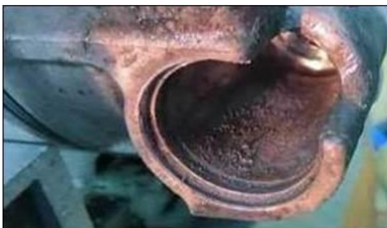
Figure 14. Corrosion in the N280 valve bore.
