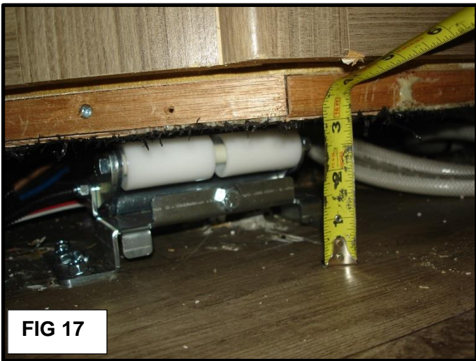
FIG 17: Once all 8 screws are secured, the roller must be elevated so the bottom of the cabinet sits exactly at 3 inches from the floor. If the roller was elevated to put screws in, you may need to lower it to the 3 inch height.
