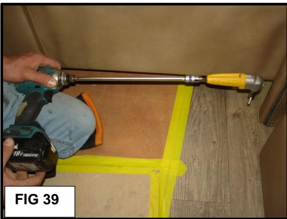
FIG 39: Use the screw gun, the extension and the right angle drill driver.
