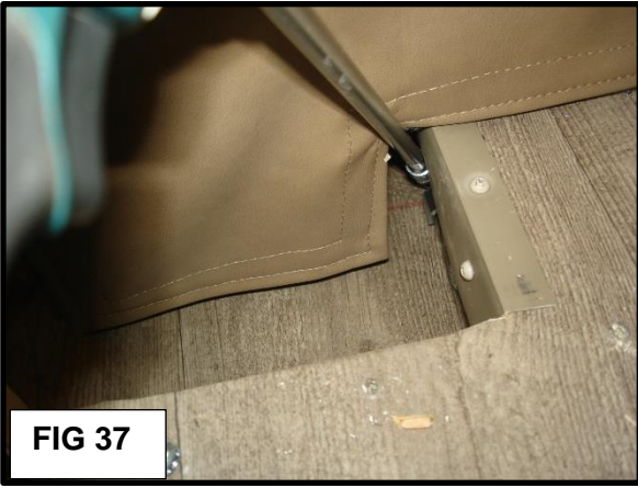
FIG 37: Use the screw gun, the long extension and the 3/8" nut driver bit. Install the front screw (closest to you) in the left / right brackets.
