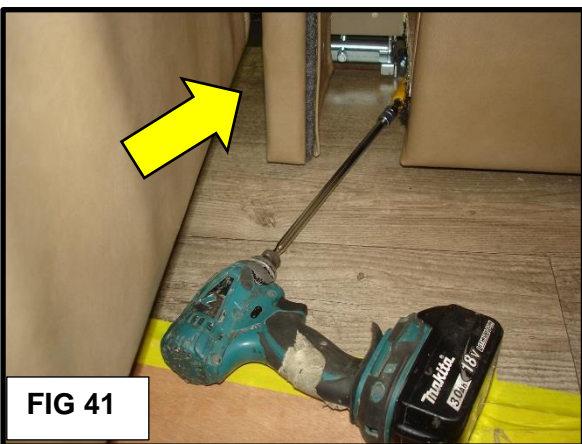
FIG 41: To install the left side screws, you need to insert the tool in the gap between the sofa and the pull out seat (arrow).
