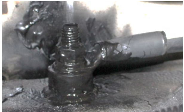
FIGURE 80: GROUND STUD WITH RUBBER COATING
