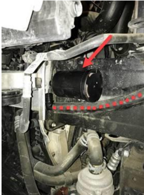
Figure 3. Installing the new NLVD filter.
