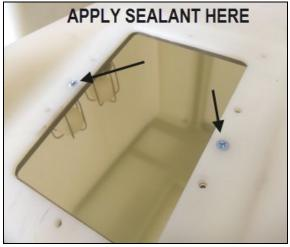
13. Install the accessory plate gasket # 032956 over the tank opening (clean both sides of the gasket with rubbing alcohol first) and install the assembled accessory plate on the tank (reuse mounting hex screws with the new supplied copper washers # 5001392; apply thread sealant on all screws).
