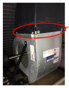
Secure the blower duct using existing hardware
