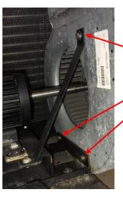
Remove and save the screws, lock washers and washers
