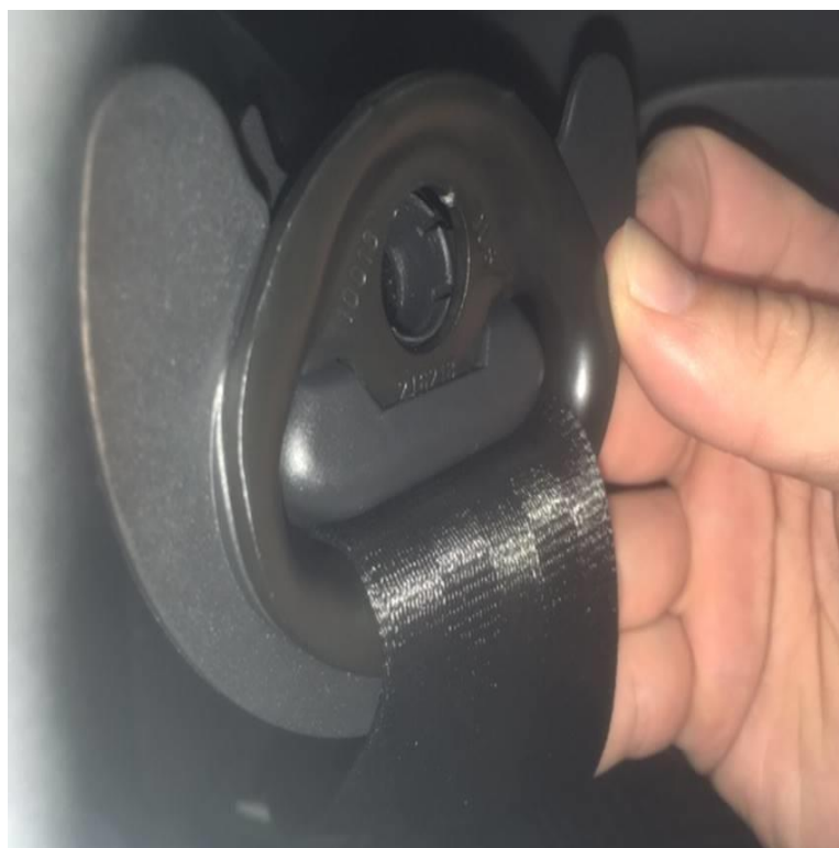
Figure 3. Removing old seat belt guide starting at the bolt hole.
