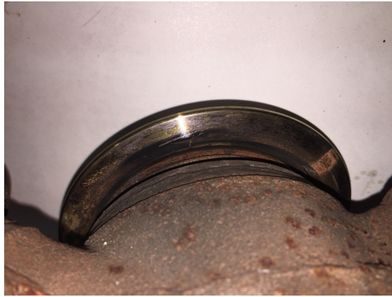
Flange weld at EGR cooler inlet
