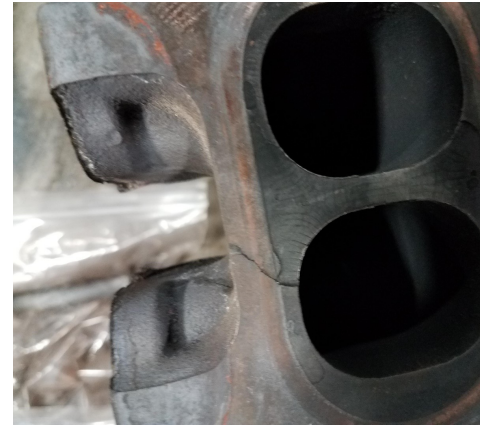
Cracks in Manifold or warped face causing leaks at gasket
