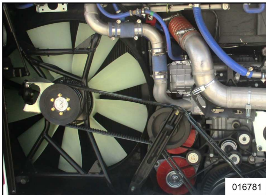
Figure 1: Cooling fan drive
