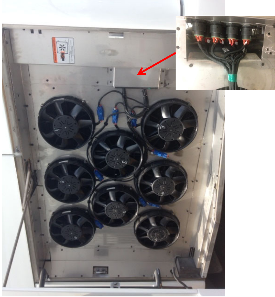
Fan and shroud installation
