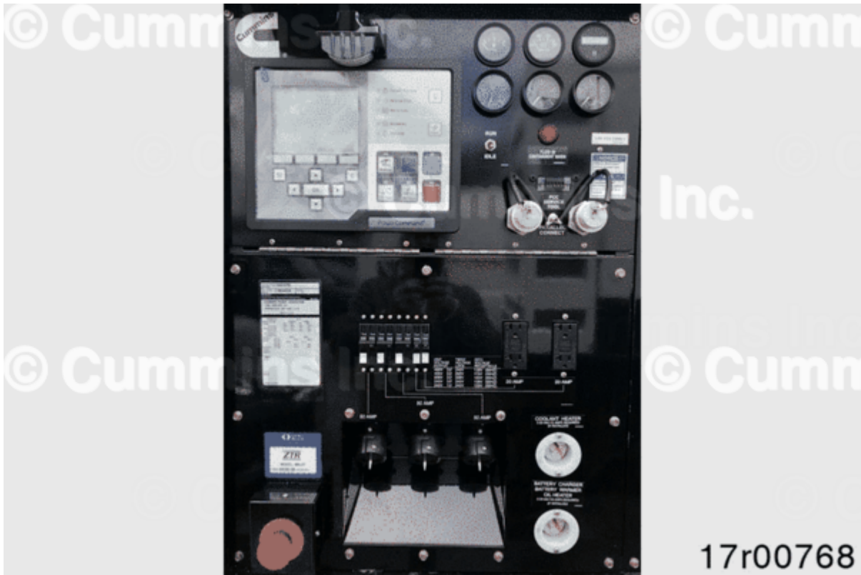
Figure 3, To access K23, open the bottom half of the panel using a 10 mm socket
