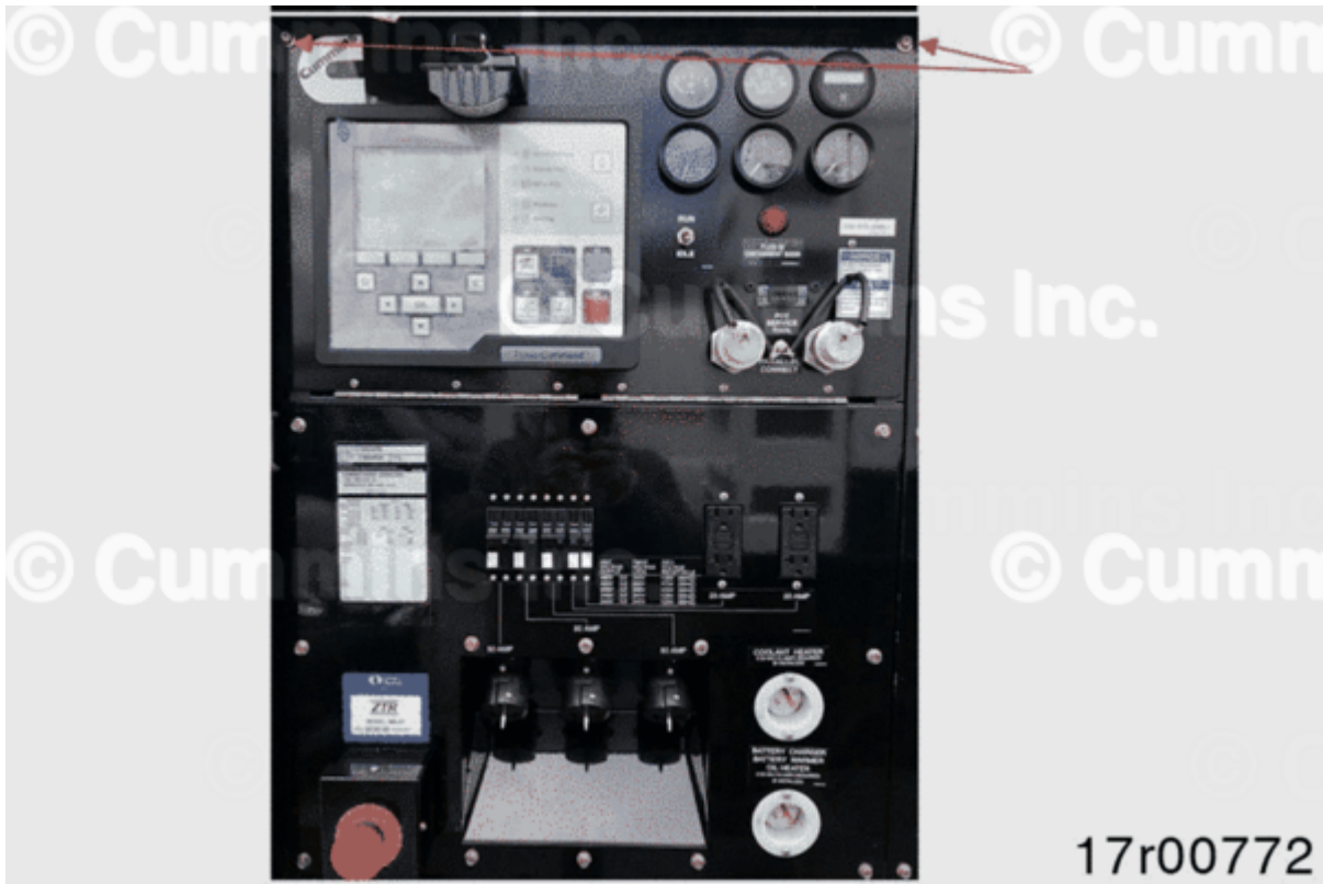
Figure 7, Open front panel by removing the two screws
