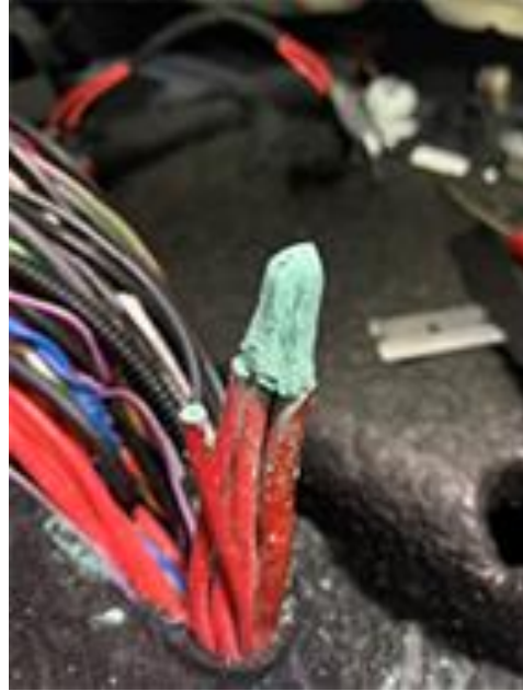
Figure 2. Close up of the wire color and damage.
