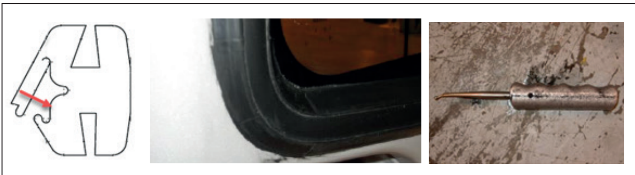
Figure 7 - Inserting the Lock
