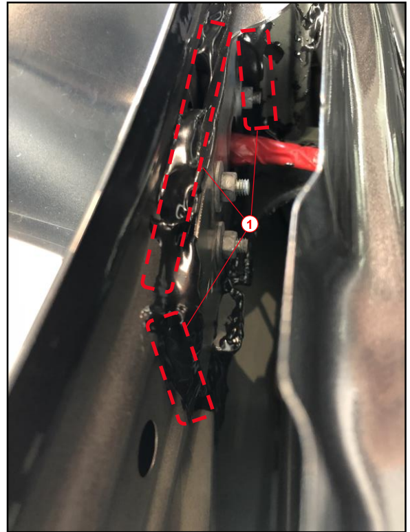
Figure 10. Completed Assembly Condition
