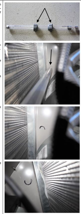
14. From the inside, drill a small pilot hole in the middle of the marks (both sides).
