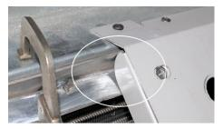
8. From the inside (using an angled drill), drill the two mounting holes in the housing (use the holes in the support tabs as a guide). Use a short **1/4 or 7/32 in (6mm)** drill bit.
