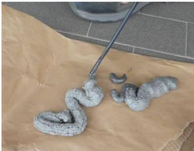
Figure 7. Purging air from the nozzle in preparation of the cavity fill.
