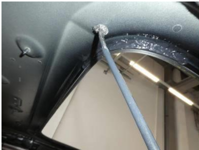
Figure 11. Filling the cavity with foam.
