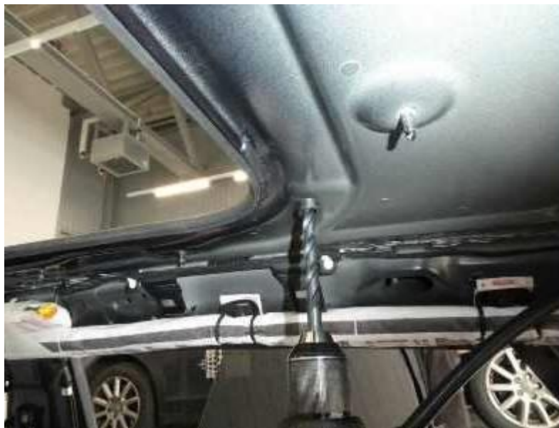
Figure 4. Drilling the 10 mm hole.
