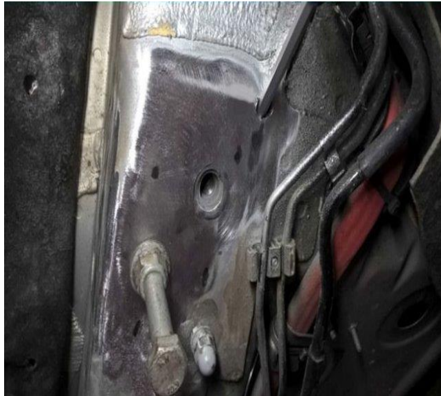
Figure 6. Bolt and nut installation.
