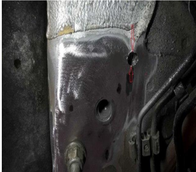
Figure 11. Access hole drilled in correct location.
