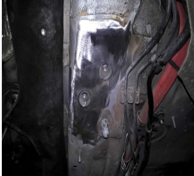
Figure 17. Weld drilled hole closed.
