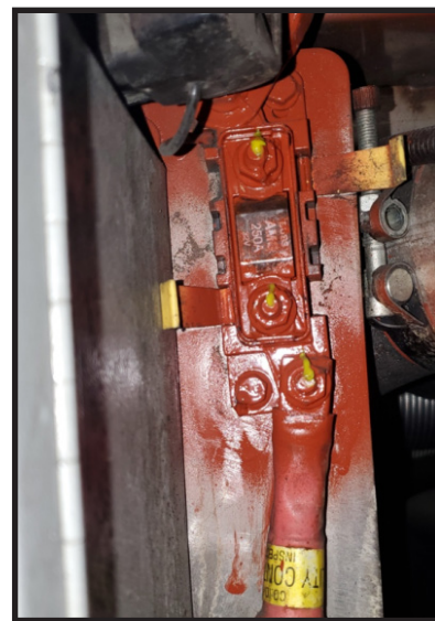
Figure 12 - Dolph ER-44 and Yellow Torque Seal Applied
