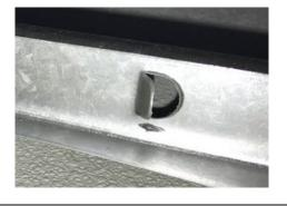
5. Insert the MERV filter in the frame rail. Take note of the airflow direction of the filter.
