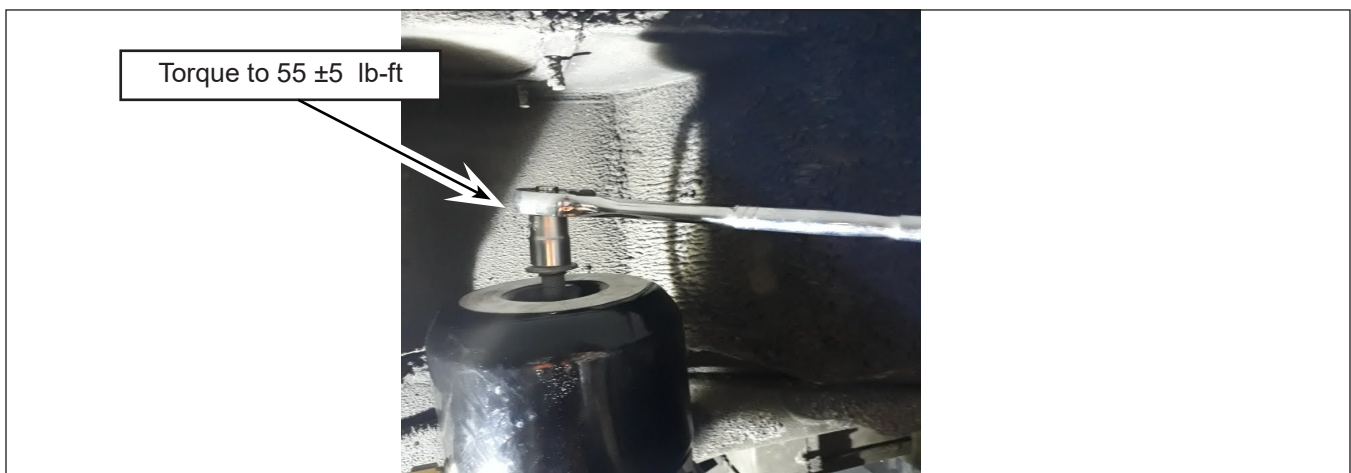
Figure 6 - Tightened the New Chamber Release Bolt
