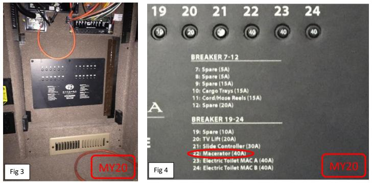
Correction for Cause #1: MY19 The breaker for the macerator in MY19 is tripped off at the DCB board on the passenger side, rear bulkhead, behind the carpeted panel shown in Fig 5-7.
