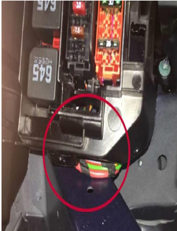
Figure 3. Area to inspect for chaffing.
