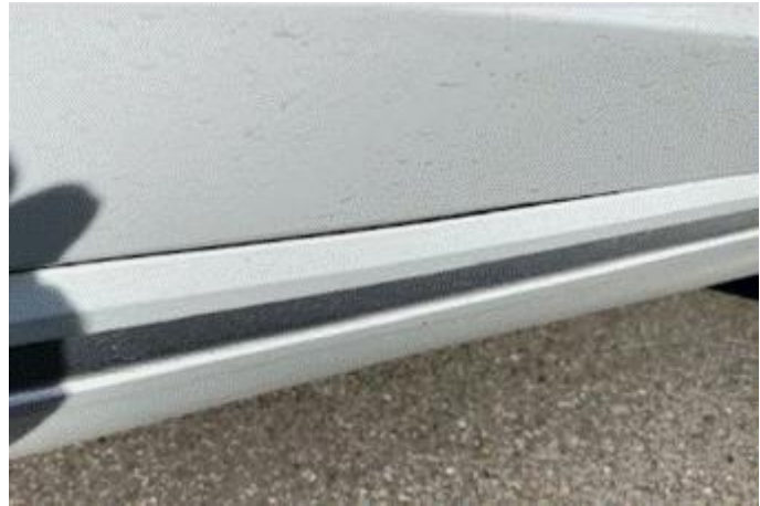
Figure 2. Closer view of the gap present between the front door trim cover and the outer door panel.
