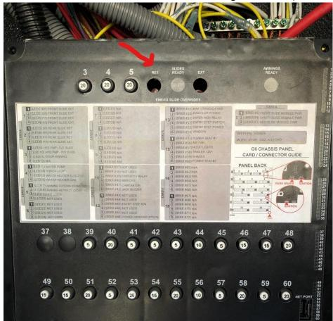
3. Place an ink pen in the "EMERG SLIDE OVERRIDES" "RET" hole. If all slides retract together, the unit is already correct and needs no further action.
