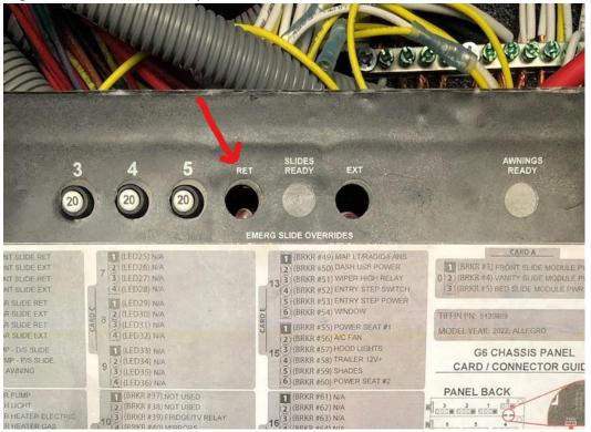
4. If all boxes retract with the exception of the bed slide, place the ink pen in the "EXT" hole at the "EMERG SLIDE OVERRIDES" location. If the bed slide then retracts, continue with the correction procedure.
