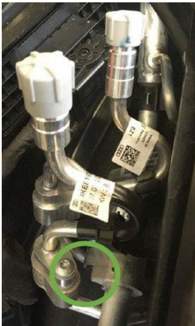
Figure 5. The refrigerant lines have been separated.
