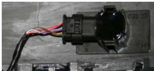
Figure 6. A correctly installed cable with sufficient length.
