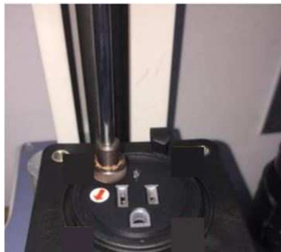
Fig. 3 Extension on AC power outlet
