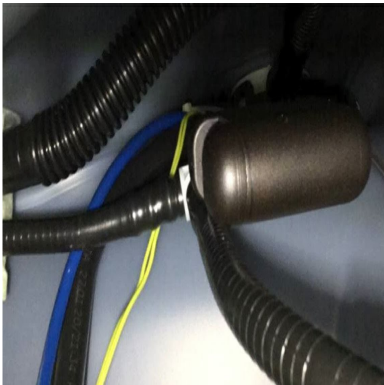
Figure 1. Checking the fuel gauge sender.
