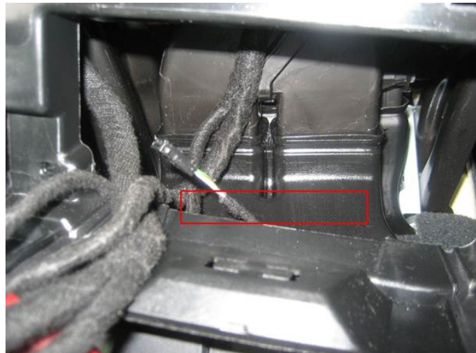
Figure 7. Mounting surface on HVAC ducting to be cleaned.
