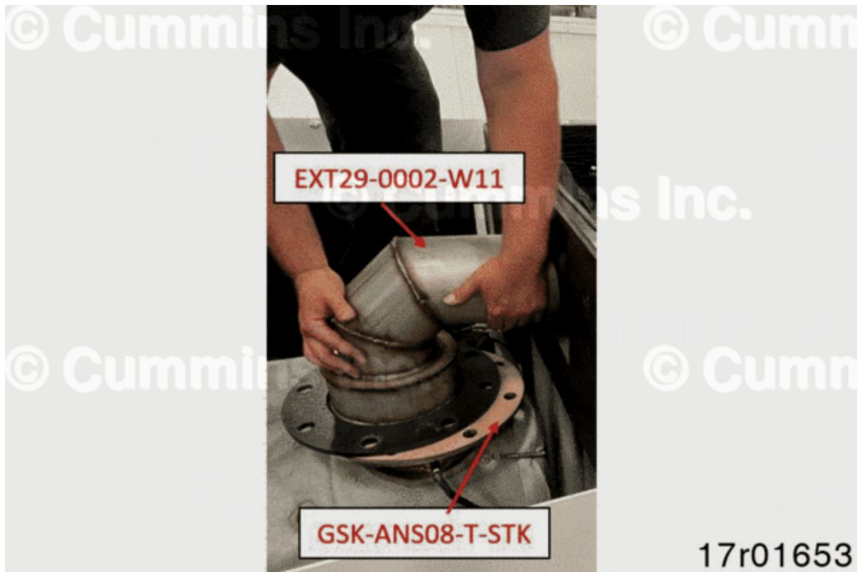
Figure 11, New Exhaust Section
