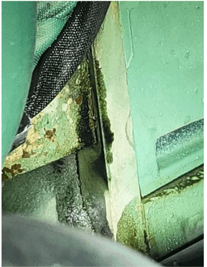
Oil actively leaking
