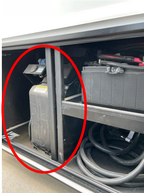
Fig. 3, DEF Tank Location
