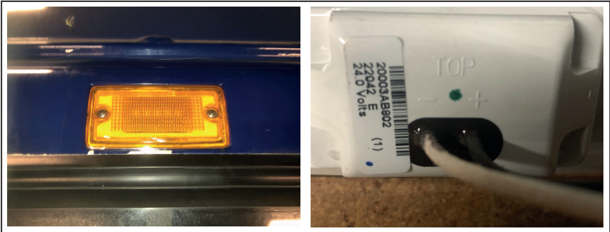
Figure 8 - Installation of marker light
