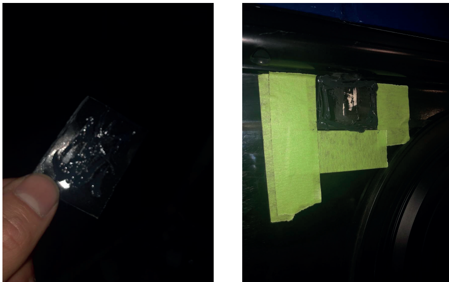
Figure 6 - Apply Adhesive
