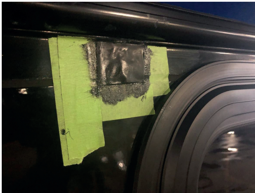
Figure 7 - Apply Tape
