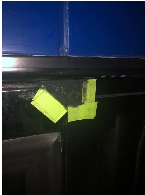
Figure 7 - Apply Tape on the Door frame
