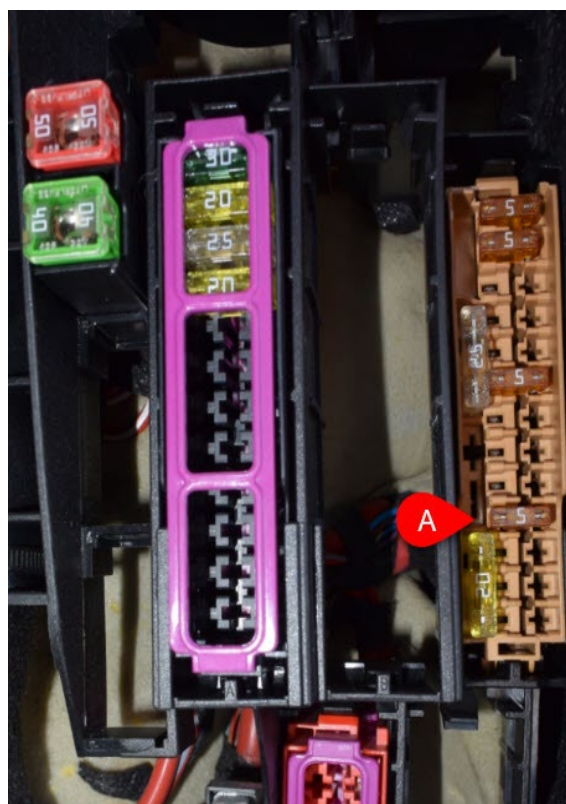
Figure 2. Fuse SF4 (5A): A4 (8W) and A5 (F5) – Left Rear Trunk.
