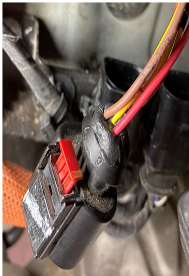
Figure 4: T6bl and T8bd butyl installed.
