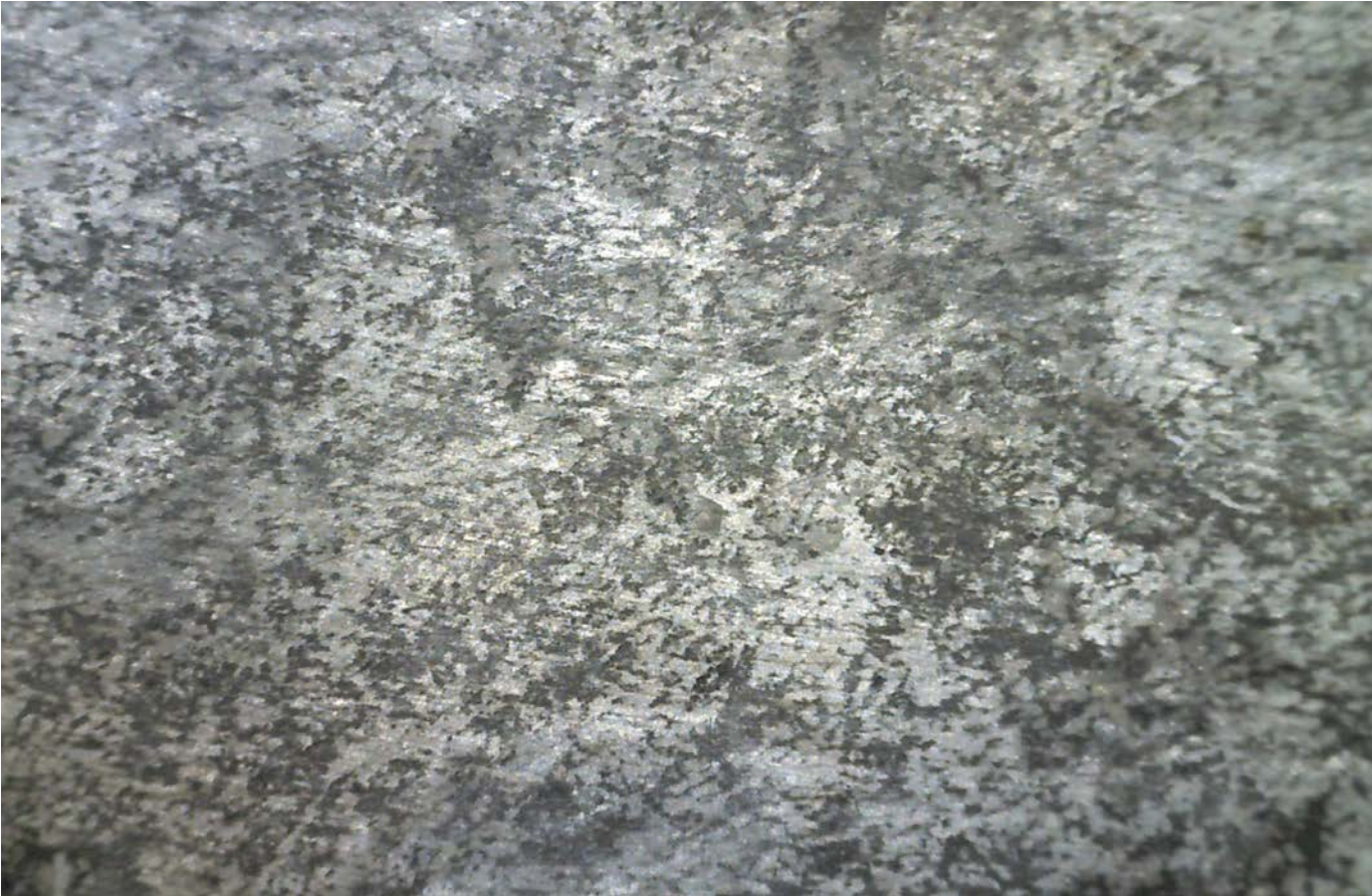
A close up of the sealing surface after cleaned with GM Low VOC Cleaner and plastic scraper.
