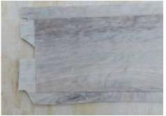
3. Apply double-sided tape to the top of the damaged section and place the replacement material on top of the taped damaged section. Ensure proper alignment and press firmly. This will keep the replacement material from shifting during the cutting process. Helpful hint: Secure the replacement material at the ends with masking tape for added security.
