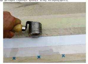
7. Remove the release liner from the seam tape and install the replacement material by starting at one side and then moving to the opposite side. To ensure a bond use a small roller over the linoleum.
