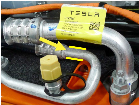
Figure 3 – Suction pipe without foam sleeve
