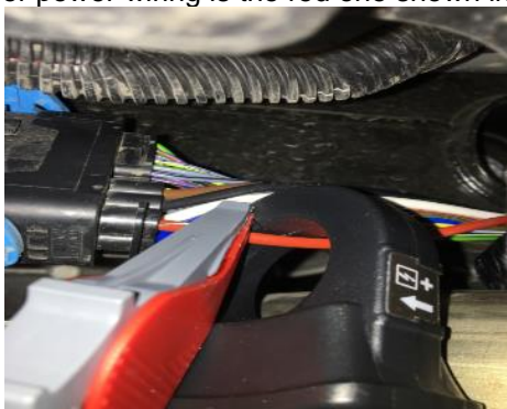
Figure 8: power supply wiring to the air suspension compressor.
