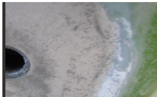
Pitting Found After Sanding Example (Fig. 1)
