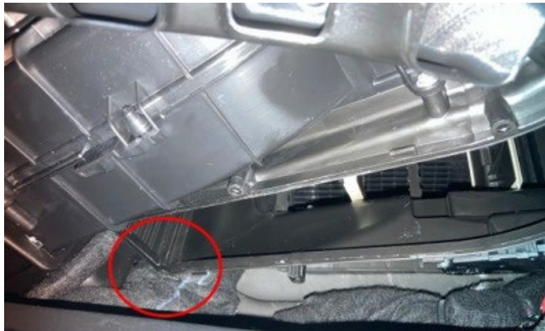
Figure 2. Interior wiring harness impingement into the dust and pollen filter cover mating surface to the air intake housing.
