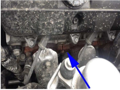
Exhaust system components
