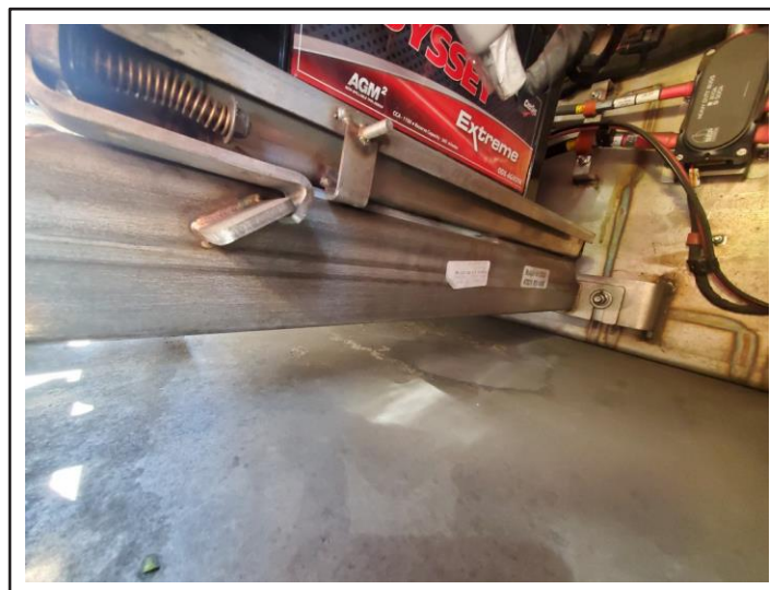
Figure 9 - Inspection of Support Arm
