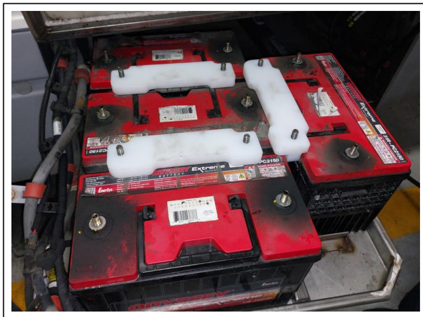
Figure 7 - Installation of Batteries and Cables
