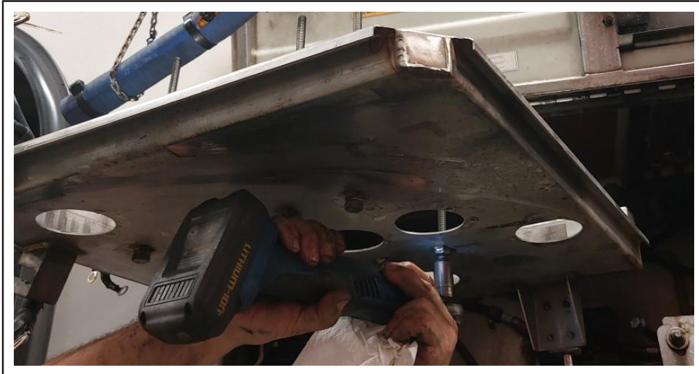
Figure 4 - Installation of Bolts Under the Tray
