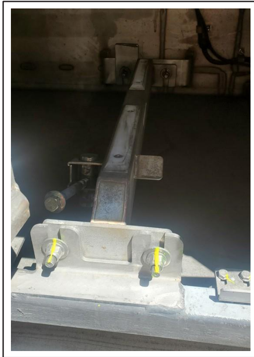
Figure 10 - Applying Torque Seal to The Nuts
