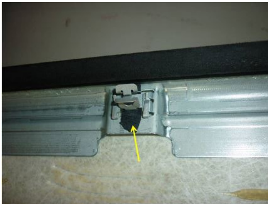
Figure 3. Clips reinstalled.
